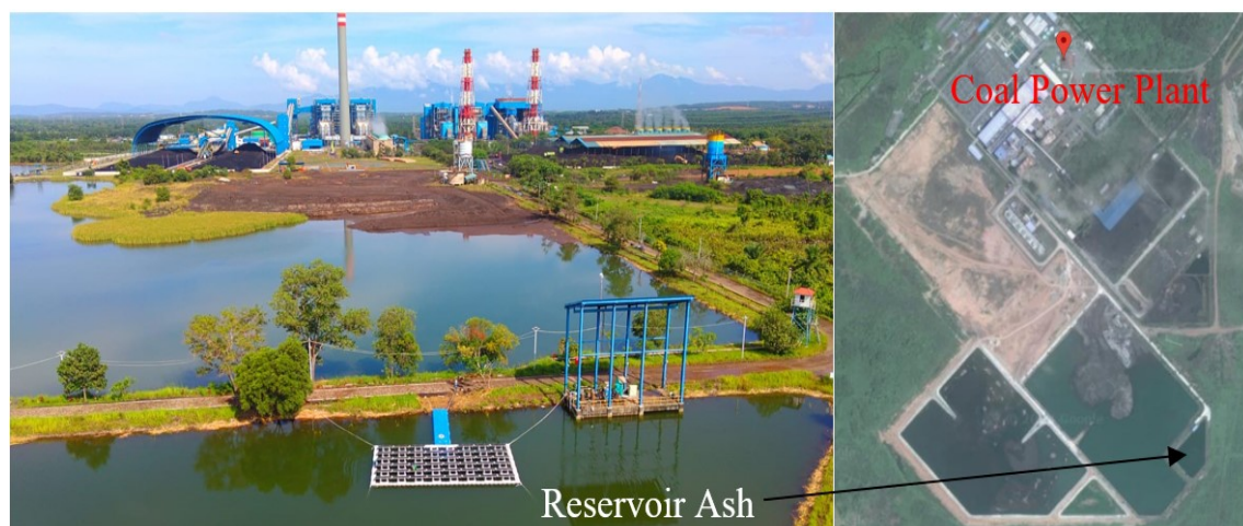
Figure 1. Floating Solar PV System on the Reservoir Ash Pond of a Coal-Fired Power Plant
