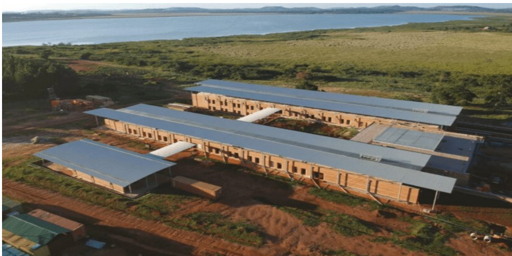
Figure 2. Renzo Piano Completes Uganda Children's Hospital with Stabilized Earth walls [4]
